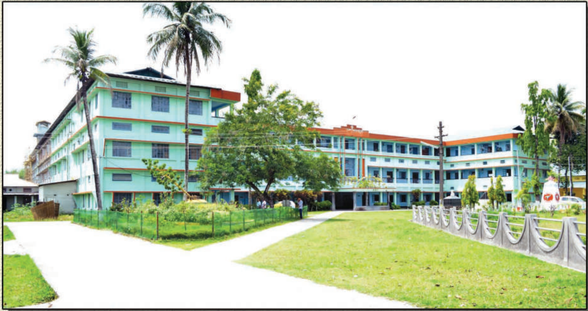
Front view of main building of the college
