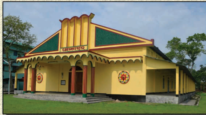
Front view of the Auditorium
